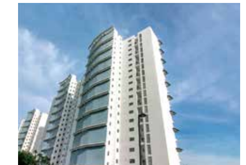
Raisina Residency Sector 59, Gurgaon 122 002. Part 1 OC Received On 29-03-2012 Part 2 OC Received On 12-12-2013 Part 3 OC Received On 01-07-2014
